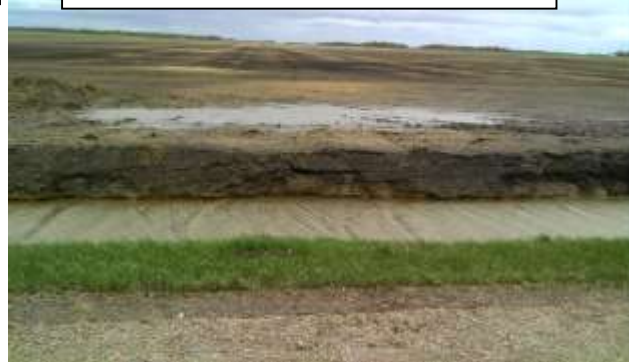
Erosion and lack of a buffer along CSAH 28, north of Trail
