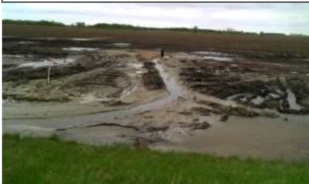
Messy well installation, north of Mentor along CSAH 12 near Beau Gerlot Creek
